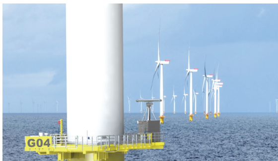
Fig. 3. Radar installation on a wind turbine tower[9]
