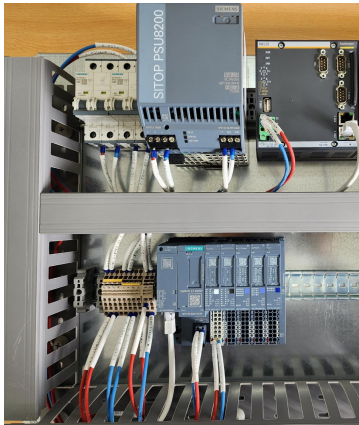
Fig. 4. Control system with MX220 PLC
