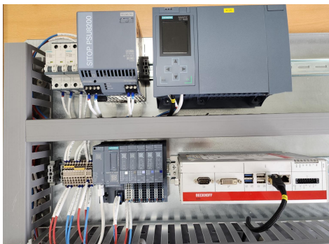
Fig. 5. Control system with S7-1500 and C6920
